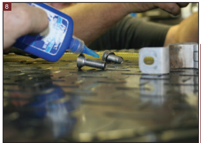
Threadlocker should be used on these bolts too.
